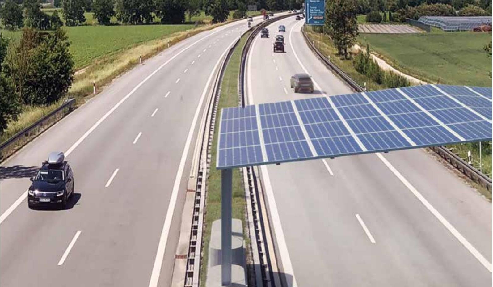
*Photovoltaic Roofing for Motorways: Concept and deployment of a demonstrator for the generation of solar energy in the road infrastructure.*
