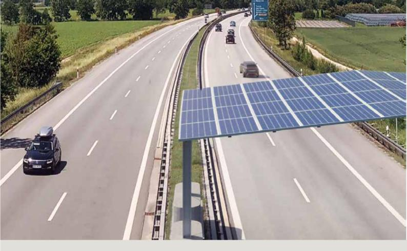
Photovoltaic Roofing for Motorways: Concept and deployment of a demonstrator for the generation of solar energy in the road infrastructure.
